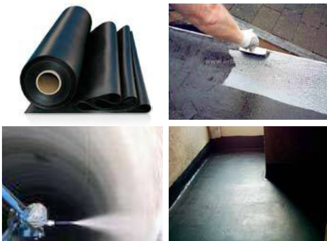
Above, from left: Waterproofing membrane, Liquid applied waterproofing, sprayed waterproofing and wet room with waterproofing before execution of finishes
